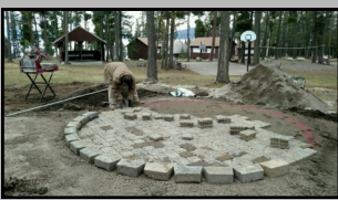
Constructing the Fire Pit
